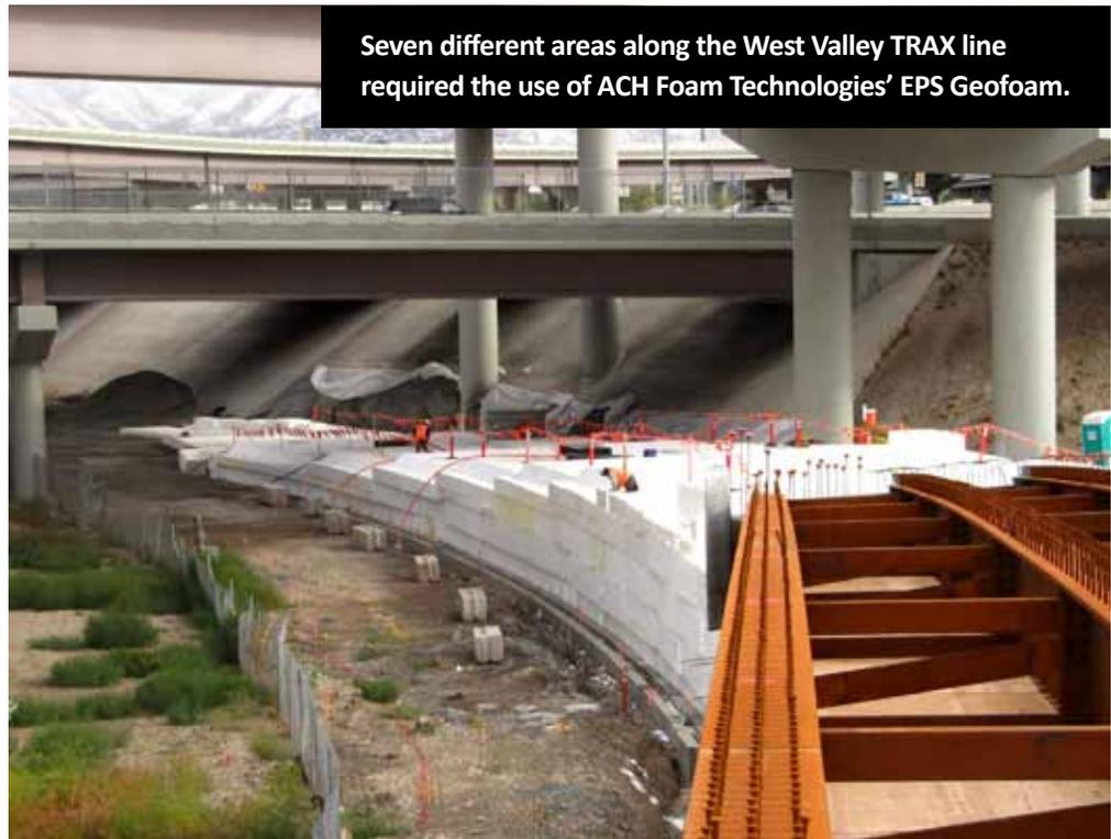
Seven different areas along the West Valley TRAX line required the use of ACH Foam Technologies' EPS Geofoam.
