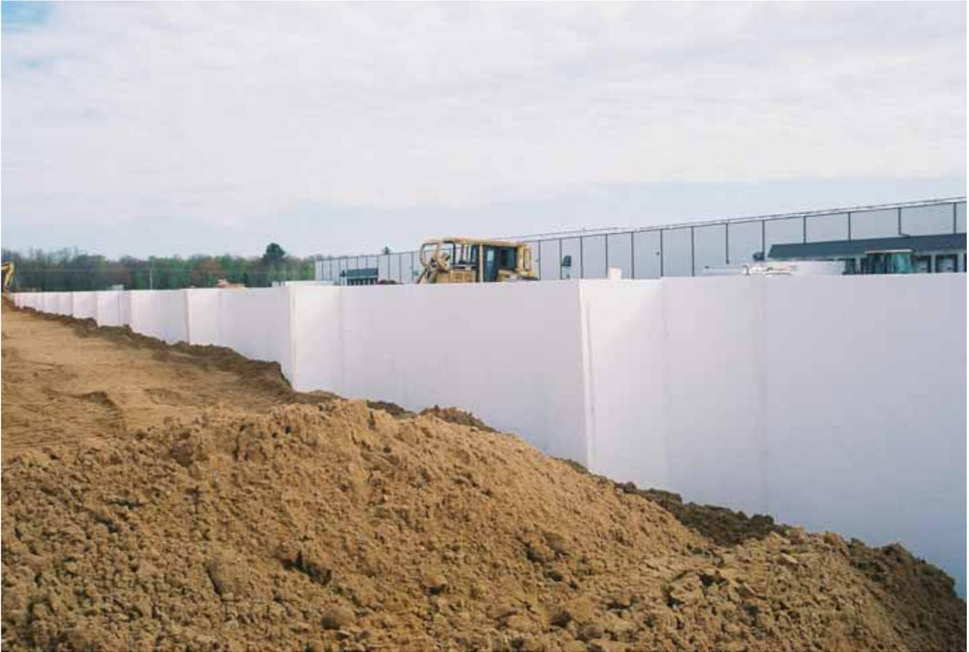
Foam-Control Plus+ architectural grade perimeter and underslab EPS insulations are designed to maintain R-value better than XPS because their permeability allows trapped moisture to escape.
