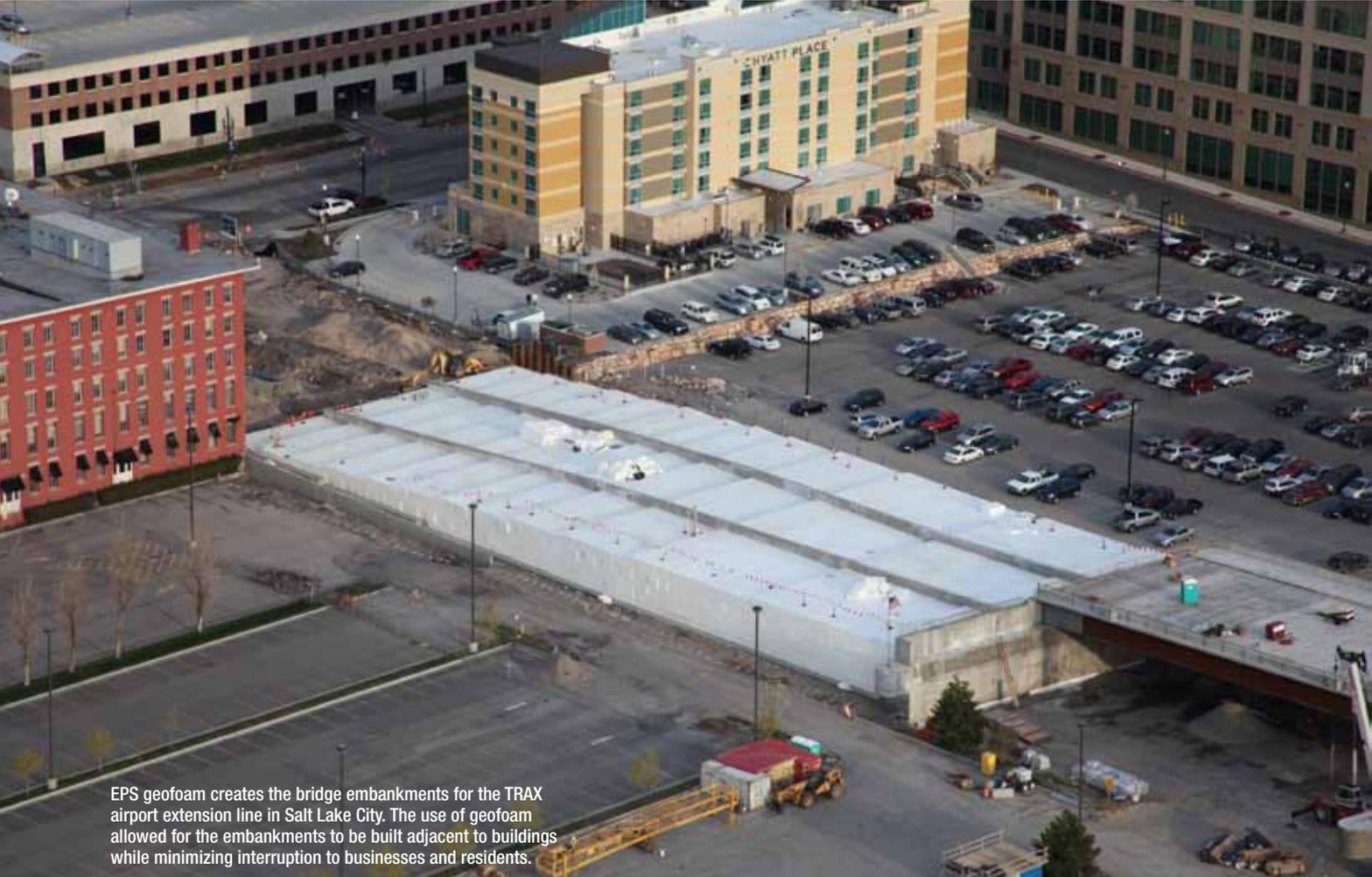
EPS geof foam creates the bridge embankments for the TRAX airport extension line in Salt Lake City. The use of geof foam allowed for the embankments to be built adjacent to buildings while minimizing interruption to businesses and residents.
